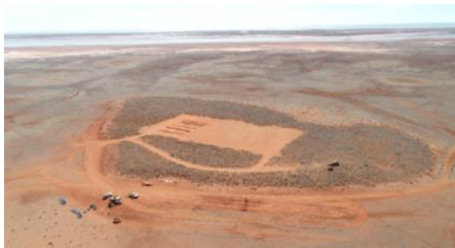
Figure 3: Small-scale Evaporation Trial Under Construction
